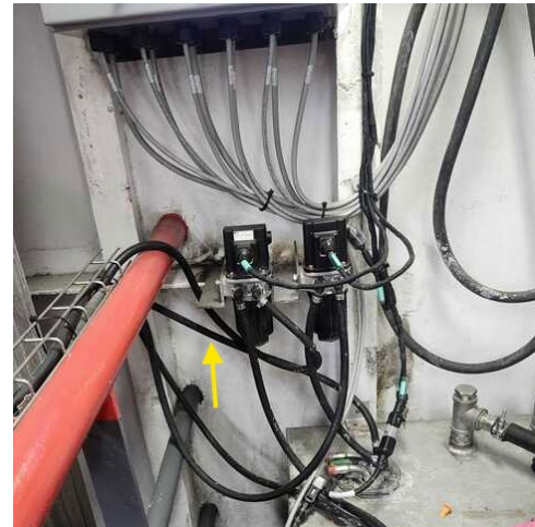
DEF hose post-repair, loop removed
